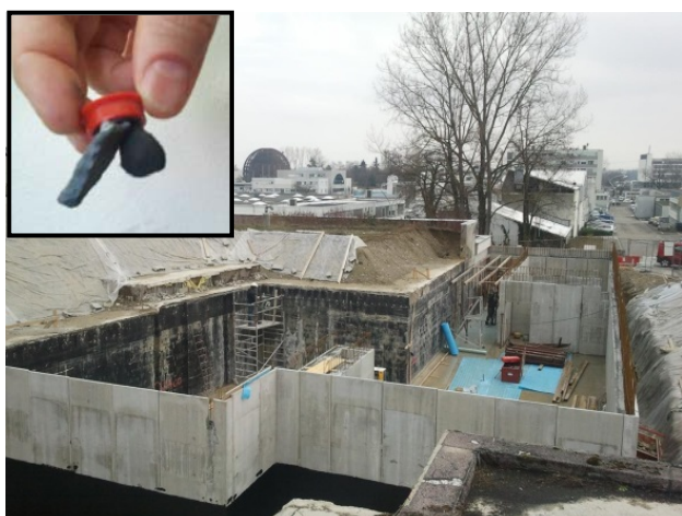
Fig. 2: Building as seen on the CERN-MEDICIS construction site, taken on February 4 th , 2014. Insert: magnetite stone and loaded cement used to make heavy concrete shielding walls (not yet to be seen on the picture).
