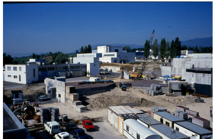
Figure 1: The ISOLDE facility during construction in 1992 [2].
