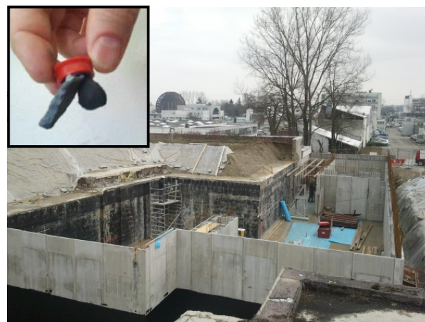
Fig. 2: Building as seen on the CERN-MEDICIS construction site, taken on February 4 th , 2014. Insert: magnetite stone and loaded cement used to make heavy concrete shielding walls (not yet to be seen on the picture).
