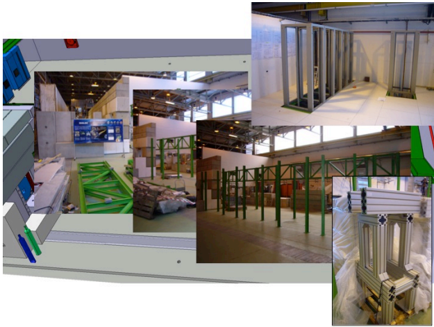
Fig.7: First stage of the HIE Linac and beamlines. HEBT carrying structure for cable trays and infrastructure being installed; HEBT cable trays and cabling installation as of April; water cooling and vacuum infrastructure as of May; HEBT elements will arrive as of September. Prioritized installation: XT00/01 to be ready by mid-Feb 2015, XT02 by mid- April 2015.
